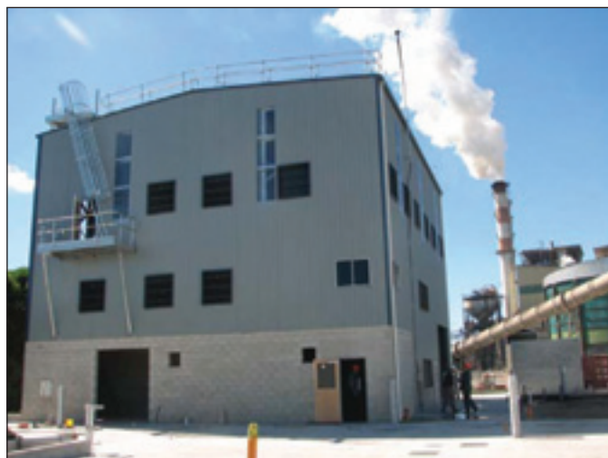
The Mackay Renewable Biocommodities Pilot Plant is a pilot scale research and development facility for the conversion of cellulosic biomass (such as sugarcane bagasse) into renewable transport fuels (bioethanol) and other high value co-products in an integrated biorefinery.
