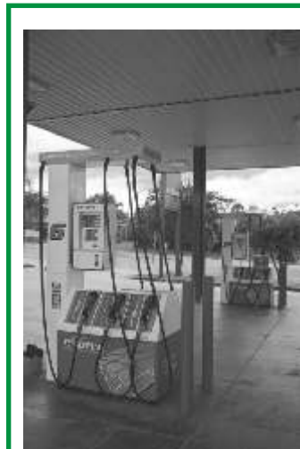
Ethanol blended fuels are available at all bowzers at the new Evolve petrol station, making the fuel readily available to consumers.
